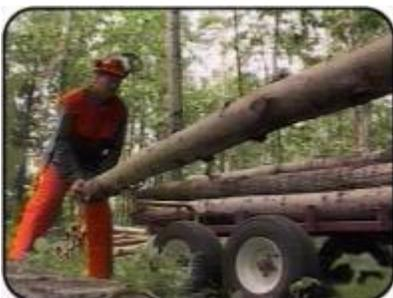
4. Position the logs against the posts on the opposite side of the trailer. This will allow you to load a maximum number of log before having to install the log posts on the pivot side.
